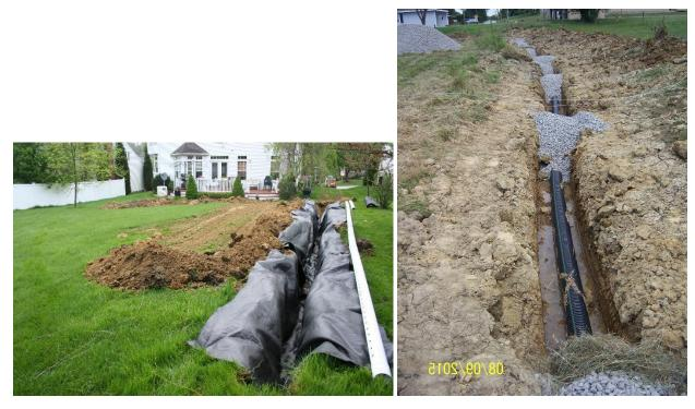
Perforated pipe covered with stone and wrapped in fabric
