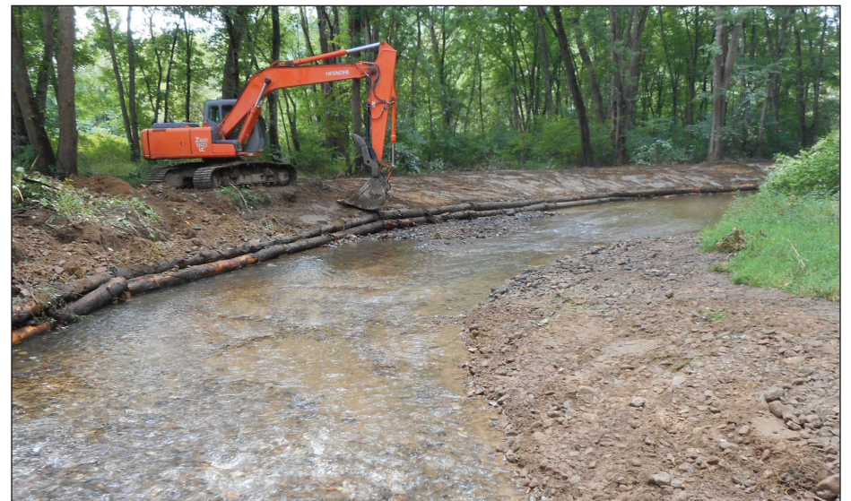
Streambank improvement project on Jacobs Creek above Bridgeport Dam
