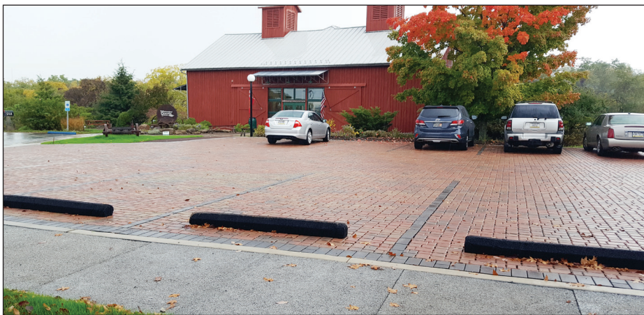
Permeable paving parking demonstration at the J.Roy Houston Conservation Center funded by Richard King Mellon Foundation, 2016.
