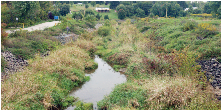
Jacobs Creek - Stream Stabilization
