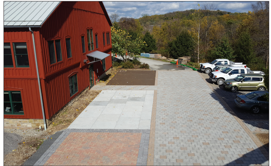
Permeable paving demonstration at J.Roy Houston Conservation Center, Greensburg, PA.
