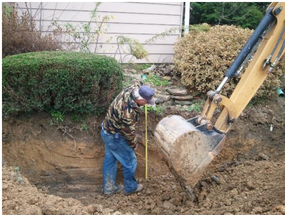
Excavate a drywell at least 10' from foundation
