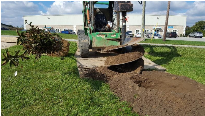
Plywood sheets protect lawn from compaction
