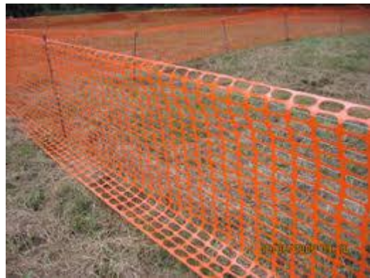
Fencing protects areas from compaction
