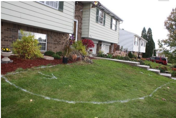
Mark rain garden location to avoid utilities
