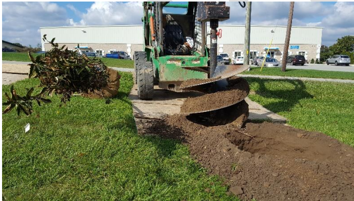
Plywood sheets protect lawn from compaction
