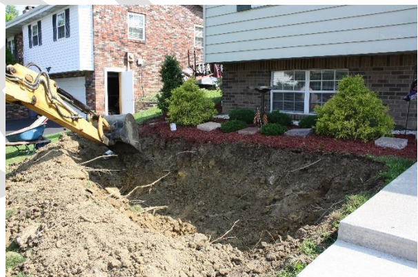
Excavate rain garden at least 10' from foundation
