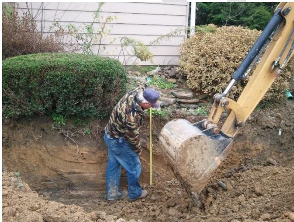
Excavate a drywell at least 10' from foundation
